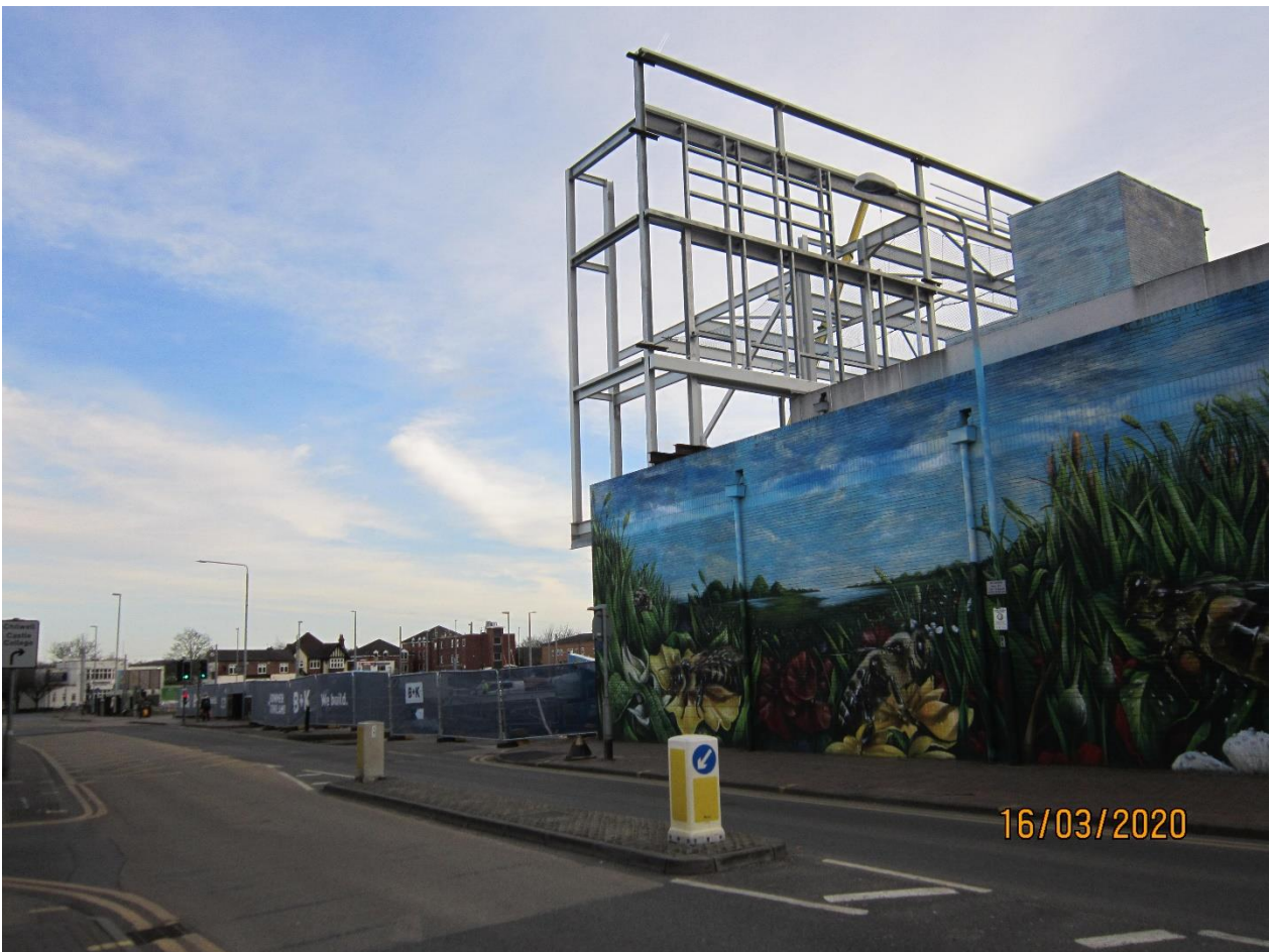
View from Station Road looking towards site and Middle Street
